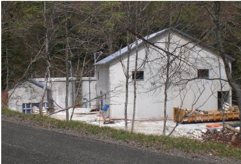
Figure 7: Example of SMBF plant in touristic site (5.000 PE)
